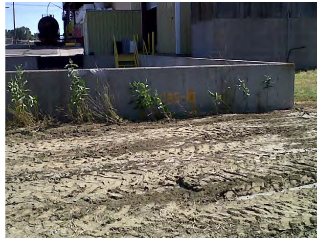
Post backfilling of excavation area.
