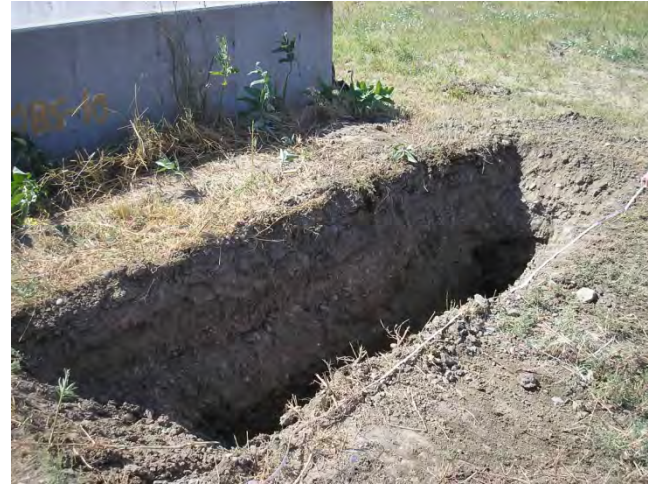
Excavation area facing southwest.
