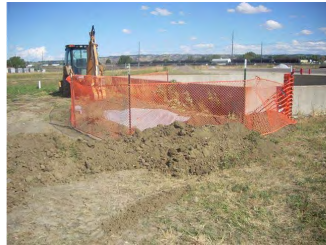
Silt fencing for access restriction and runoff.
