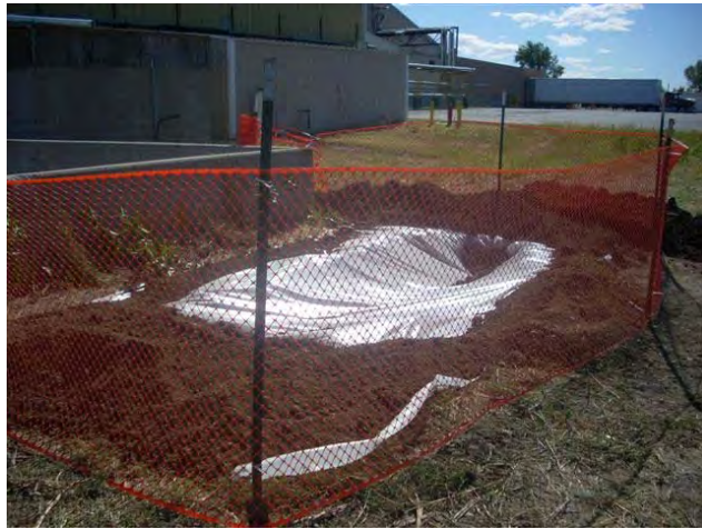
Silt fencing for access restriction and runoff.
