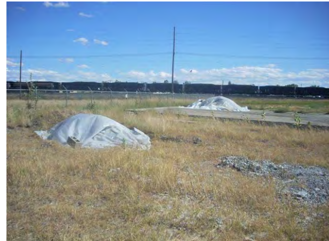
Covered soil stockpiles.
