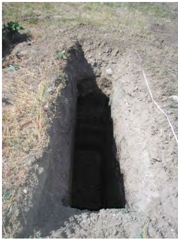
Excavation area facing west.
